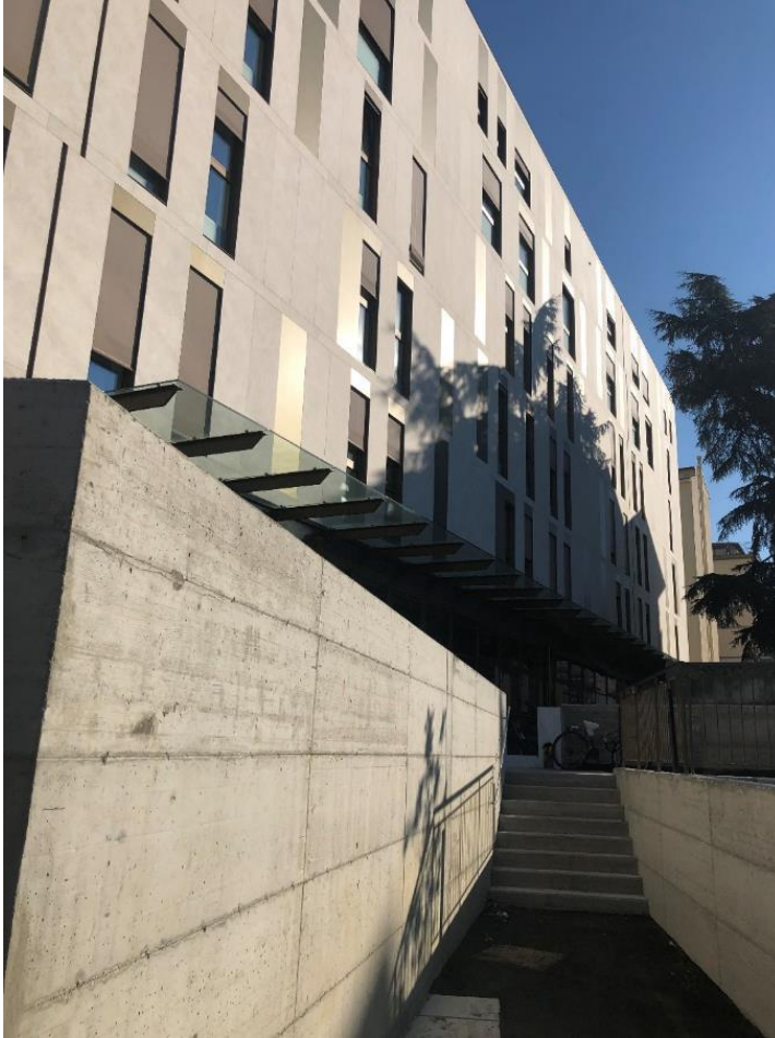
Figure 10| Camplus University Residence in Florence. Credits: TESIS archive.
